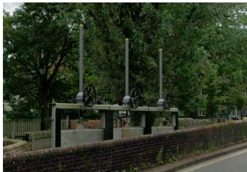
Durngate flood defenses
